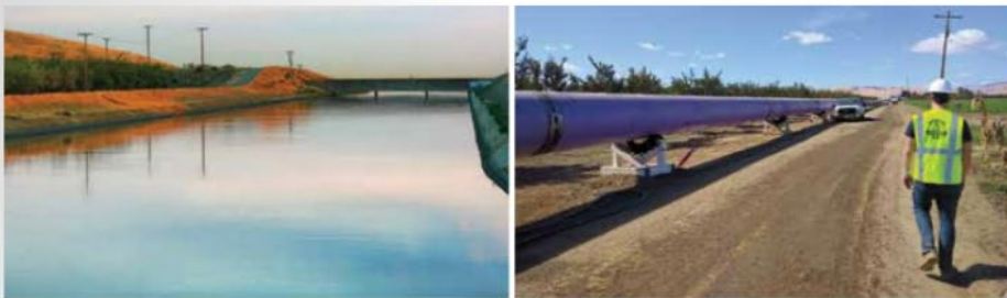
In partnership with the cities of Modesto and Turlock, Del Puerto Water District has delivered tertiary recycled water to California's agricultural lands since 2017
