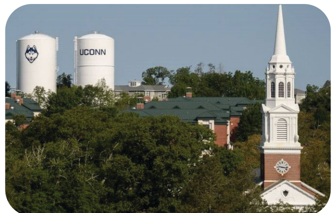
University Water Towers
