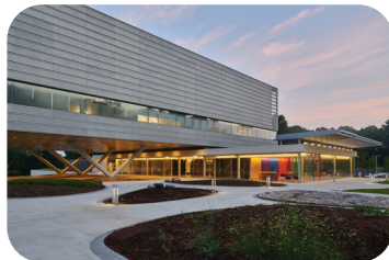
Innovative Partnership Building on Discovery Drive
