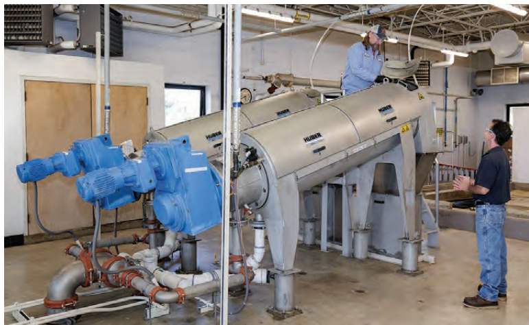
The plant's two Q-PRESS screw presses (HUBER Technology) yield cake at 17-19% solids.
