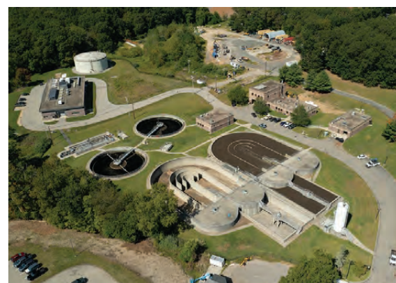
The UCONN Water Resource Recovery Facility has a design dry-weather capacity of 3 mgd, and average flows of 1.3 mgd during the school year and 0.75 mgd during summer.
