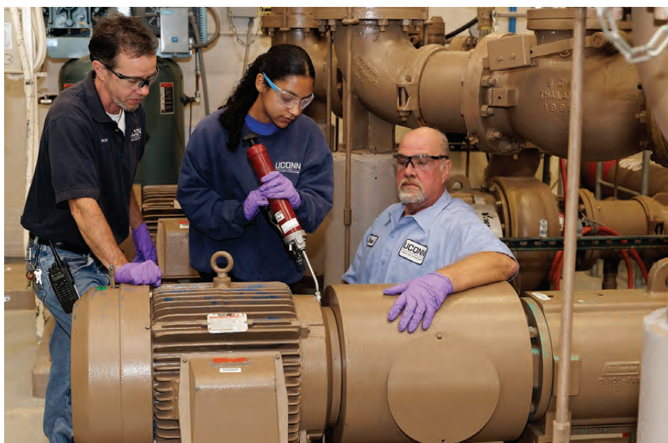
Savage, student intern Valerie Berrios Torres and operator Brian Delventhal perform motor maintenance on return activated sludge pumps (Vaughan).
